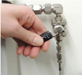
Partly open the Isolation Valve
