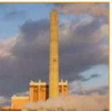
Monitoring of emissions from incinerators is a demanding application for Continuous Emission Monitoring Systems. Their emissions are highly corrosive, some of the gases are soluble and, because the waste being burnt is constantly changing, the resulting stack gas temperature varies widely.
